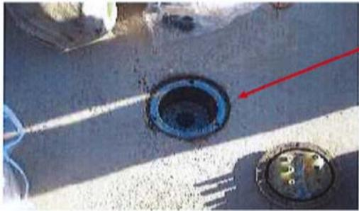
A threaded pipe plug or mechanical plug may be used to prevent water from running back into the pipe after having been drained and cleared.
