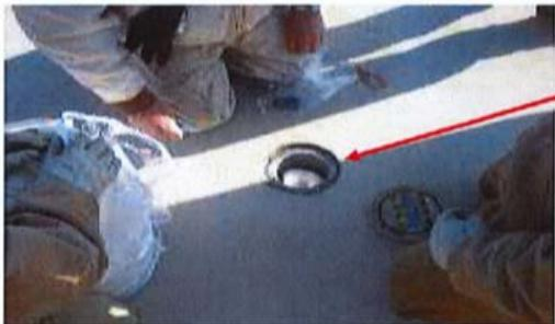
To prevent freeze expansion that could cause the can to swell and damage to concrete or the can to split, install a piece of mattress foam or Styrofoam. A 3" square is the right size for most cans.
