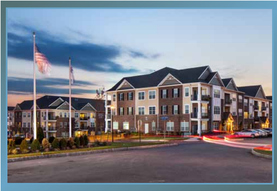
Stone Bridge at Raritan
