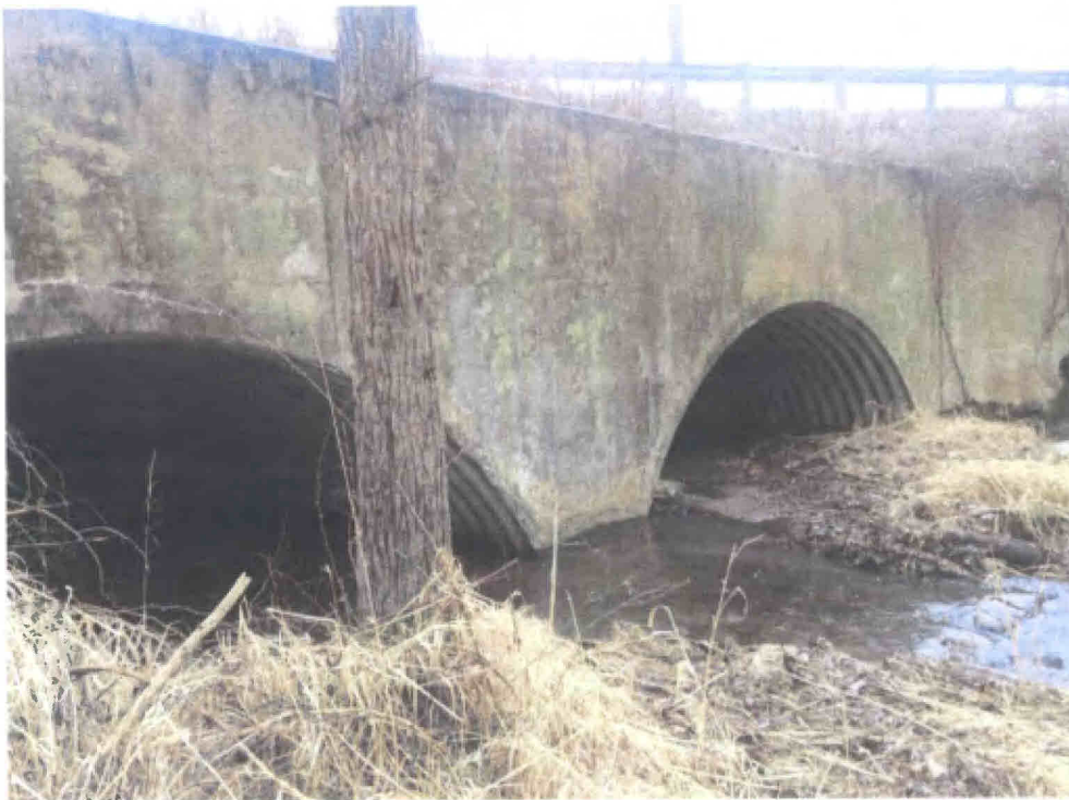
Photo 2 – North Elevation, looking southwest
