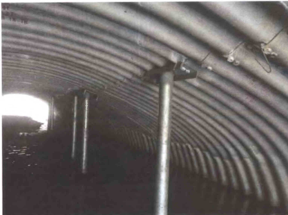
Photo 4 – East Span, looking north
