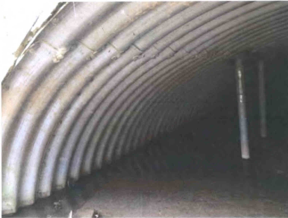
Photo 7 – West Span, looking southeast
