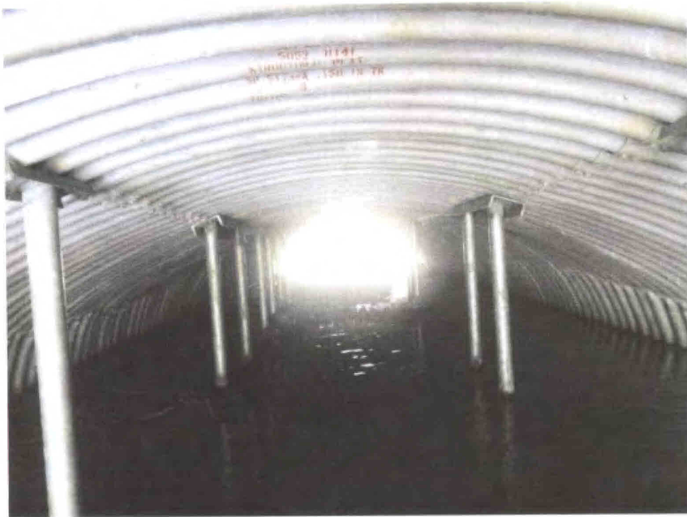
Photo 3 – East Span, looking north
