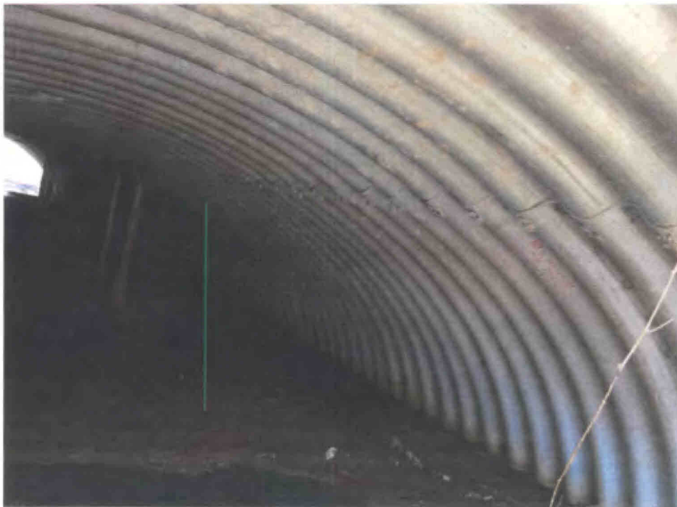
Photo 8 – West Span, looking southwest
