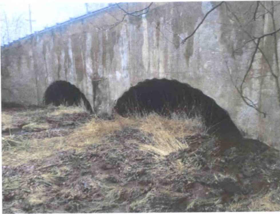
Photo 1 – South Elevation, looking northwest
