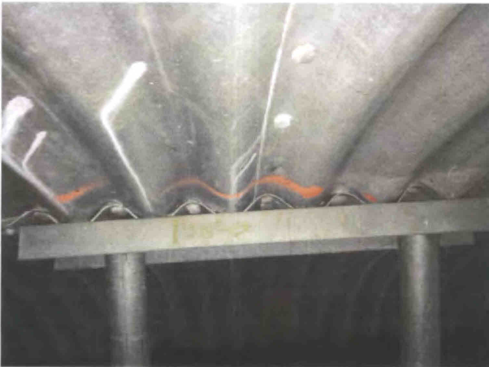
Photo 10 – West span, typical repair/shoring post
