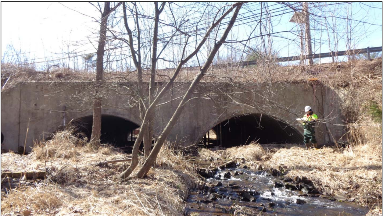
Photo No. 6: Downstream elevation view of bridge.
