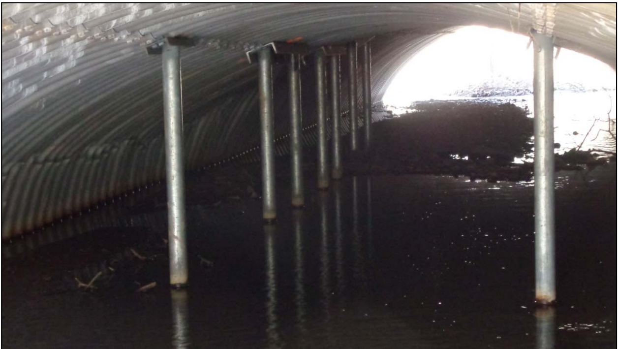
Photo No. 8: View looking downstream through east arch. Note temporary shoring.
