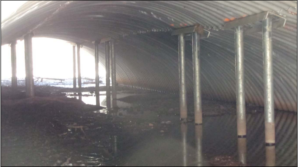
Photo No. 7: View looking downstream through west arch. Note temporary shoring.
