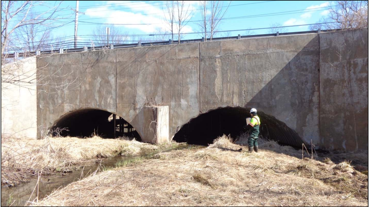
Photo No. 5: Upstream elevation view of bridge.
