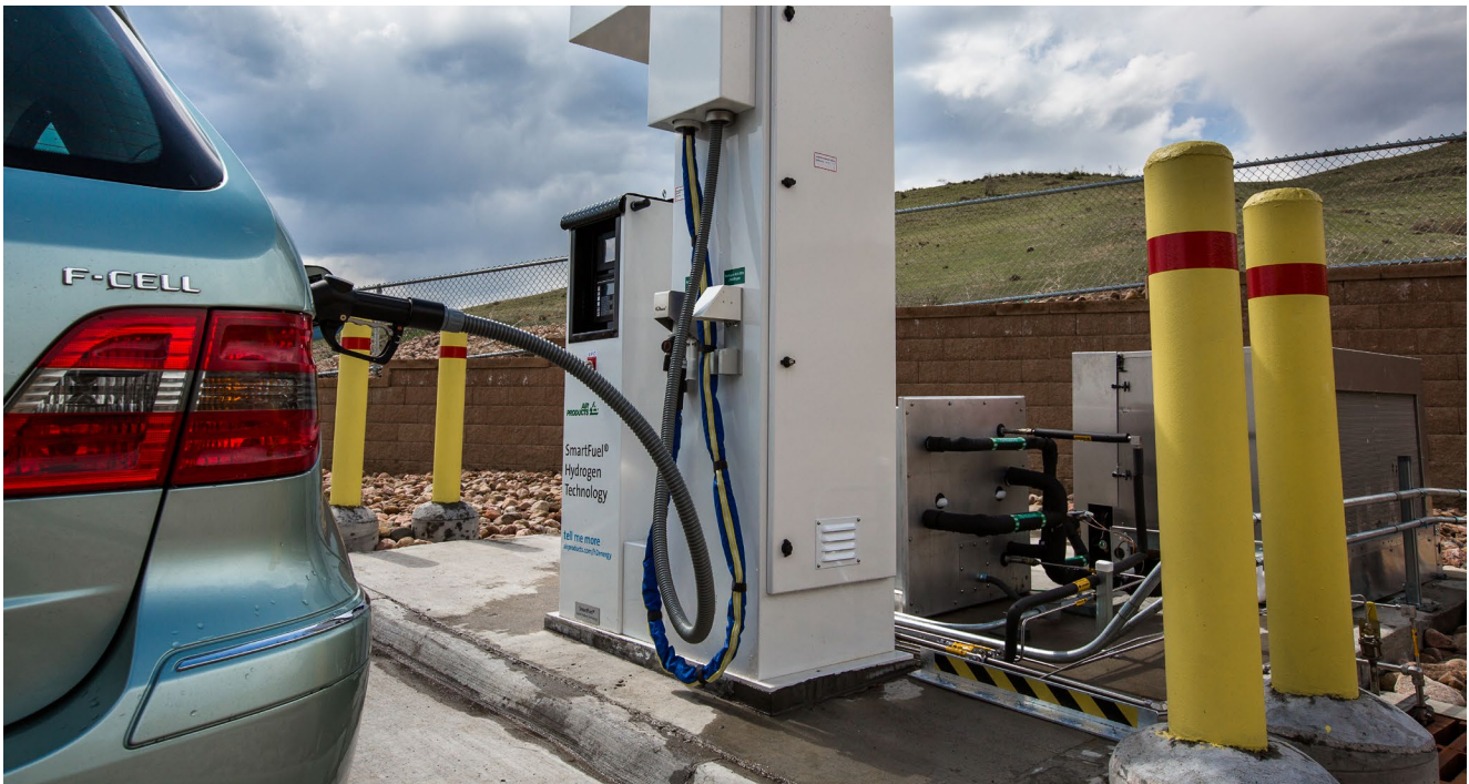
Photo by John De La Rosa, NREL 34236
