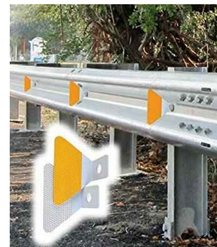
G. GUIDERAIL AND RETROREFLECTIVE DELINEATORS
