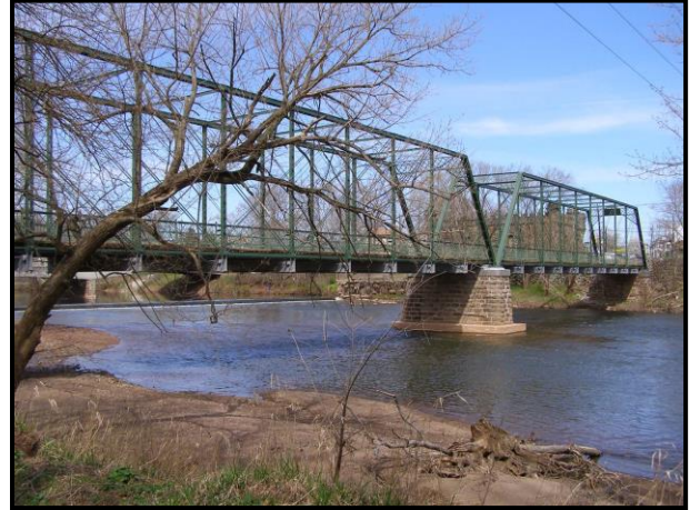
Nevius Street Bridge
