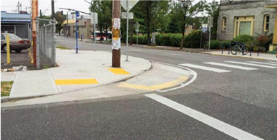
Mountable Curbs at Route 27 and Hamilton Street Intersections
