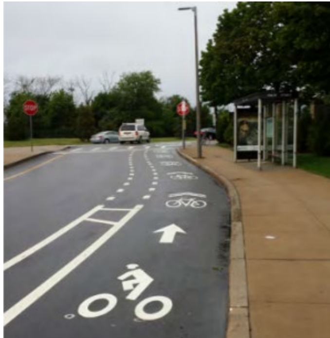
Figure 19 – Transition from Bike Lane to Shared Bus Stop Area in Boston, Massachusetts 24
