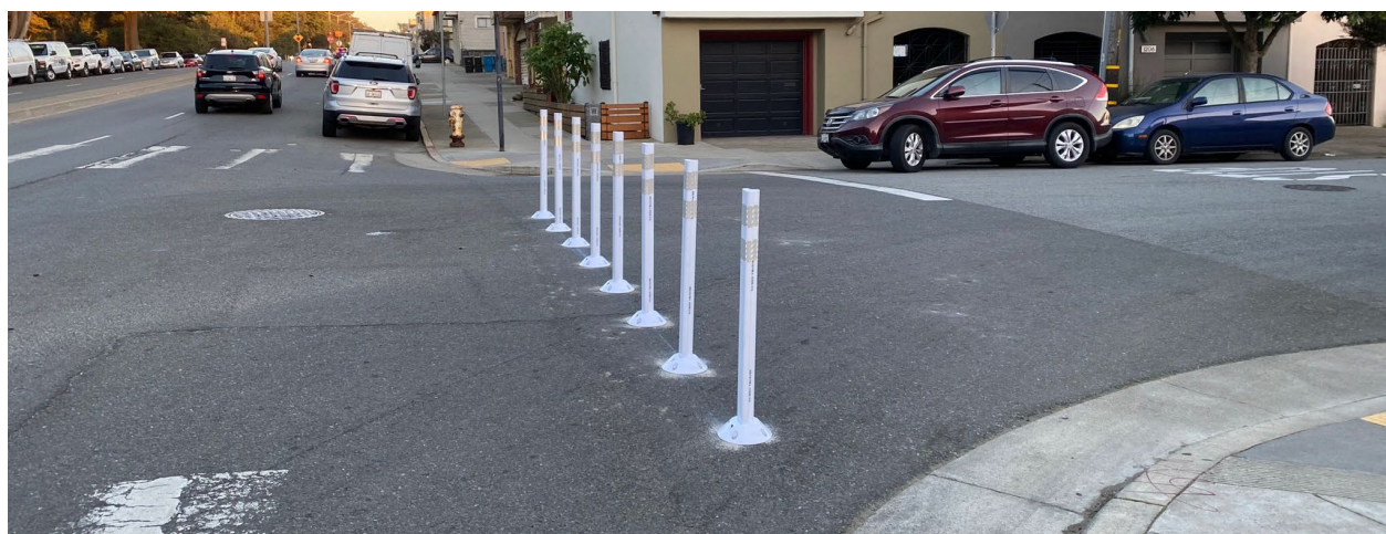
Figure 15 – Temporary Traffic Diverter Allowing Right Turns onto Main Road 16
