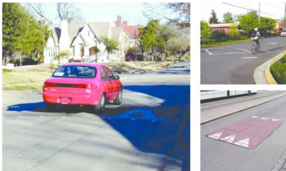
Figure 24 – Sample Speed Humps from NACTO 30
