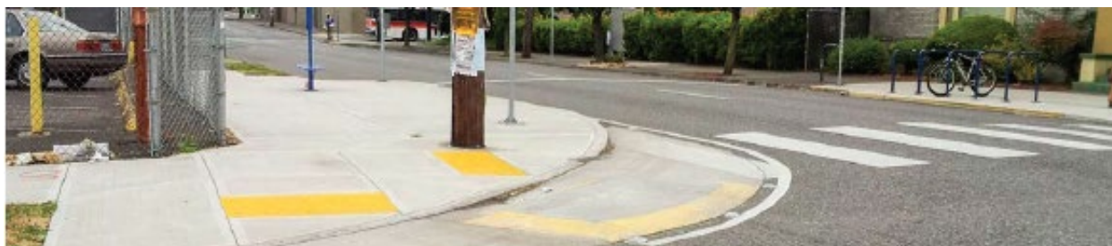
Figure 21 – Mountable Concrete Curbs in Portland Oregon 27
