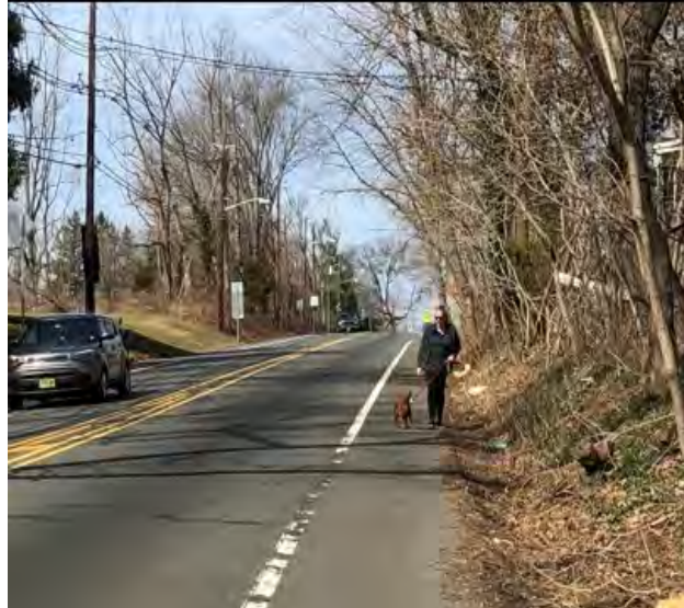
Gaps in pedestrian connectivity and pavement drop-offs on side of road
