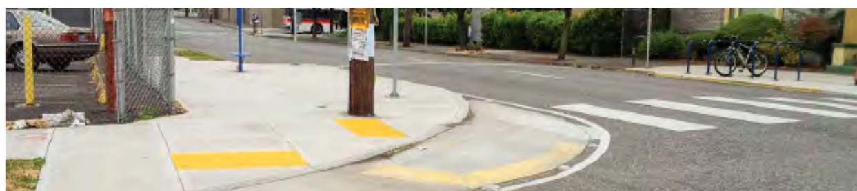
Figure 21 – Mountable Concrete Curbs in Portland Oregon 27
