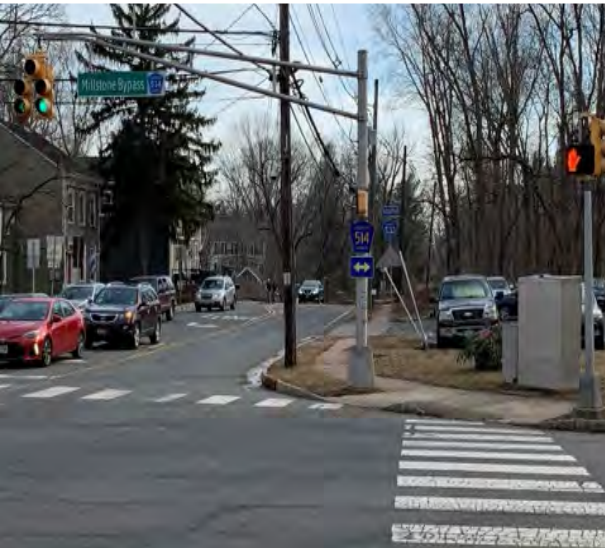
Signal at Amwell Road & Main Street lacks pedestrian countdown signal heads
