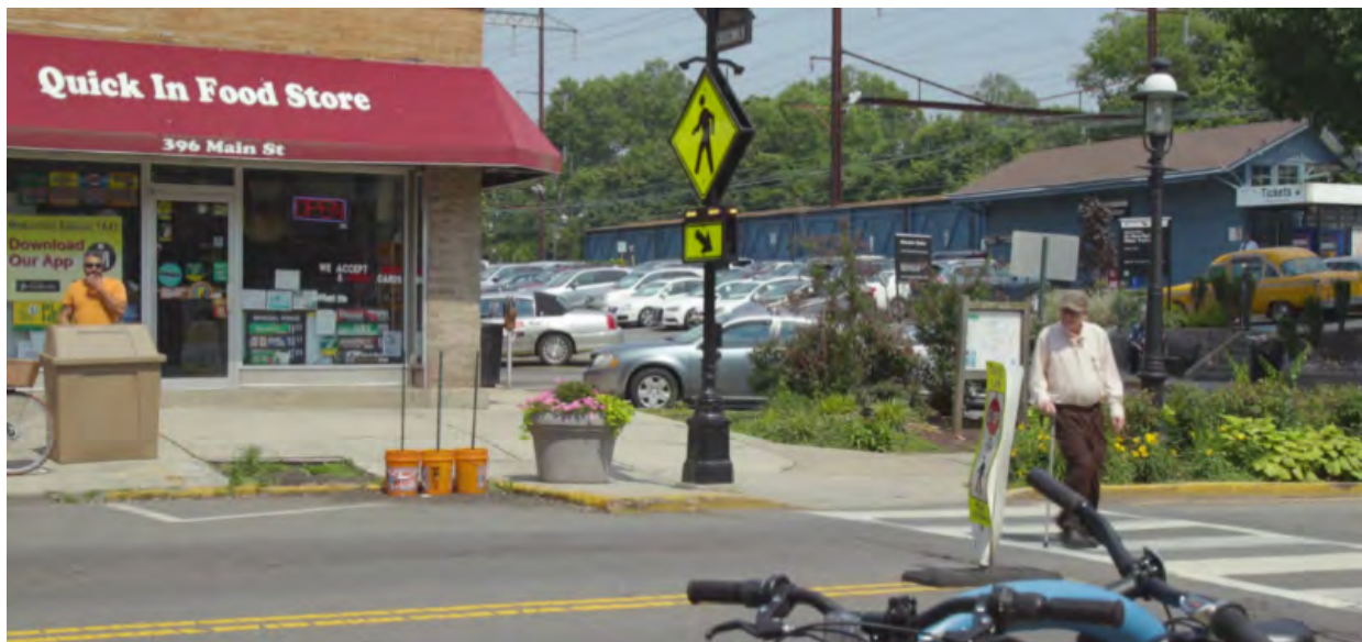
Figure 17 – RRFB Installation in Metuchen Borough by Middlesex County 27
