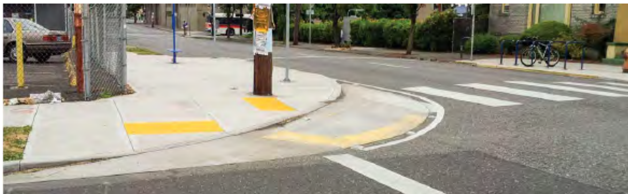
Figure 20 – Mountable Concrete Curbs in Portland Oregon 25
