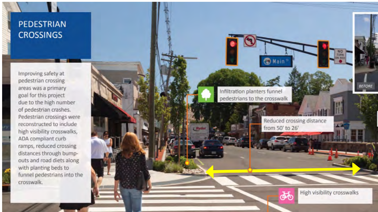
Figure 18 – Millburn Township Curb Extensions with Infiltration Planters, Details Included 25
