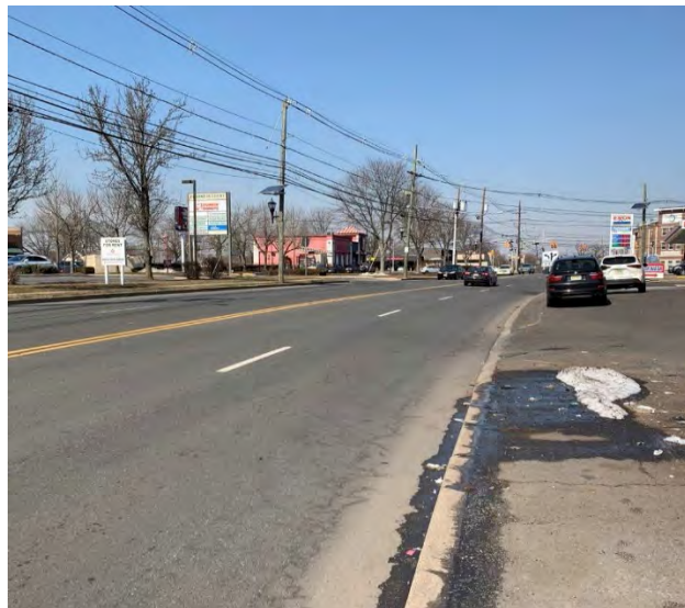
Sidewalk interrupted by wide curb cuts and vehicles encroaching on pedestrian paths
