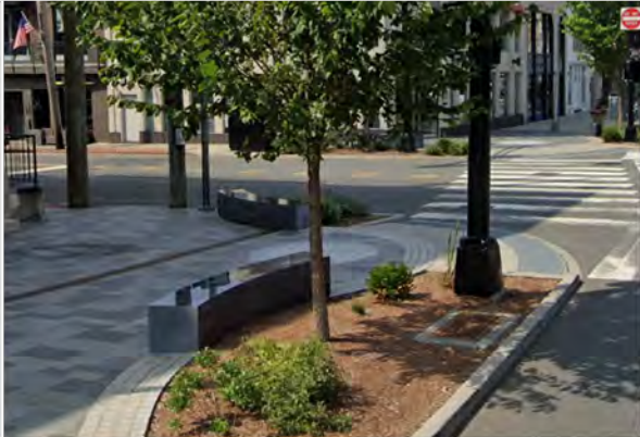
Figure 18 – Millburn Township Curb Extensions with Infiltration Planters, Details Included 23
