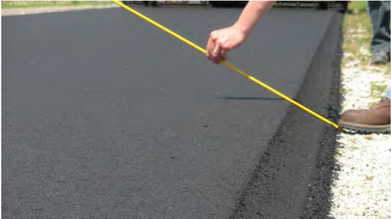
Figure 16 – Safety Edge Paving Example 23
