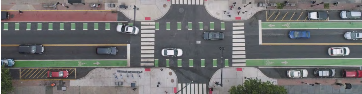
Figure 16 – Curb Extensions in the City of Hoboken 21
