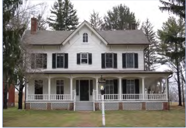
The confluence of Peapack Brook and the North Branch of the Raritan River became a rural industrial center during the 18th century when a saw mill, grist mill, tannery, and bark mill were located nearby. The Peapack Brook Rural Industrial Historic District, eligible for the National Register, includes five houses, several outbuildings and mill structures that reflect the industrial and agricultural development of the area, ca. 1750-1900. Shown here is Elm Cottage, a mid-18th-century residence with extensive mid-19th-century additions and alterations. (Photo courtesy Somerset County Cultural & Heritage Commission)
