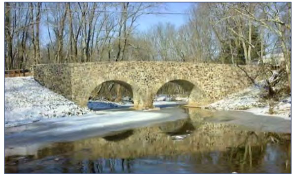
Opossum Road Bridge, Montgomery Township, over Bedens Brook, tributary to the Millstone River. Built in 1822, this bridge is among the earliest surviving in Somerset County and is listed in the National Register. The county features a number of early bridges thanks to its natural resources, for multiple reasons: the many streams with terrain unfavorable to fording for wagons, and the wealth built from farming excellent soils in a well-watered climate. (Photo courtesy Somerset County Cultural & Heritage Commission)
