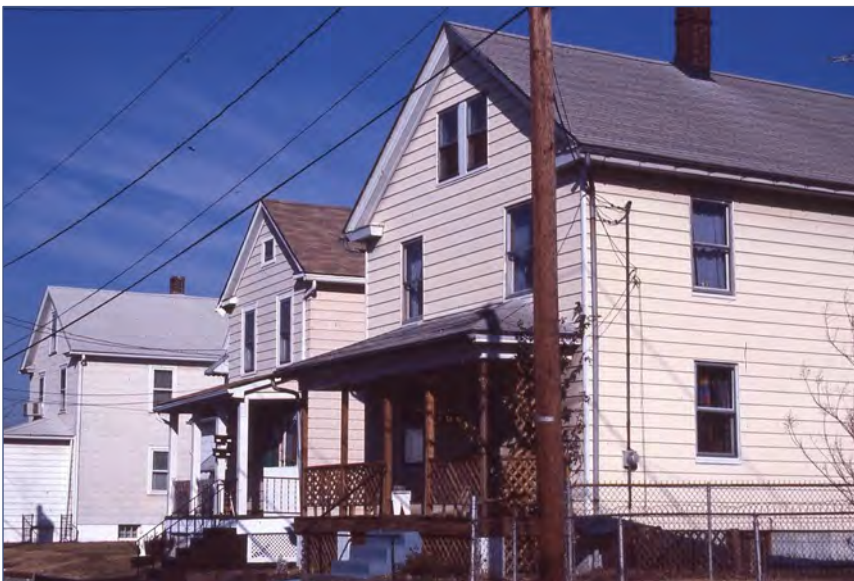
An image from a color slide made of the streetscape of Rosalie Street in Manville for the SCC&HC's six-volume historic resources survey of 1989. The form of these simple workers' houses dates from the nineteenth century and reflects the Greek Revival style with its front-facing pedimented gable - a useful style for narrow city lots. (SCCRS 18-11-4 Streetscape North side of Rosalie)
