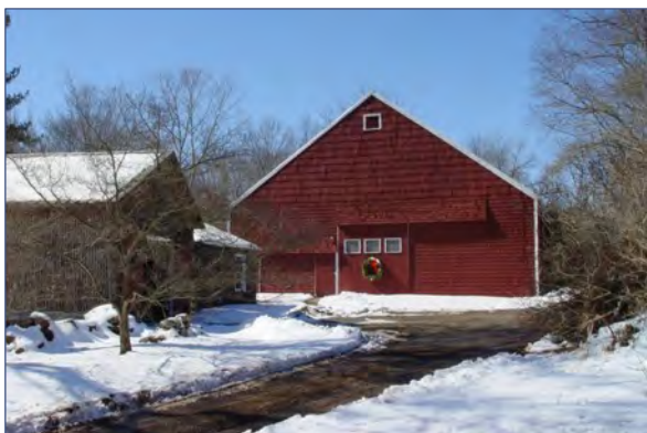
The Van Doren Barn in the Millstone River valley (c. 1755), displaying the distinctive broad gable end of a Dutch-built barn. (Photo by Ron and Pat Morris)
