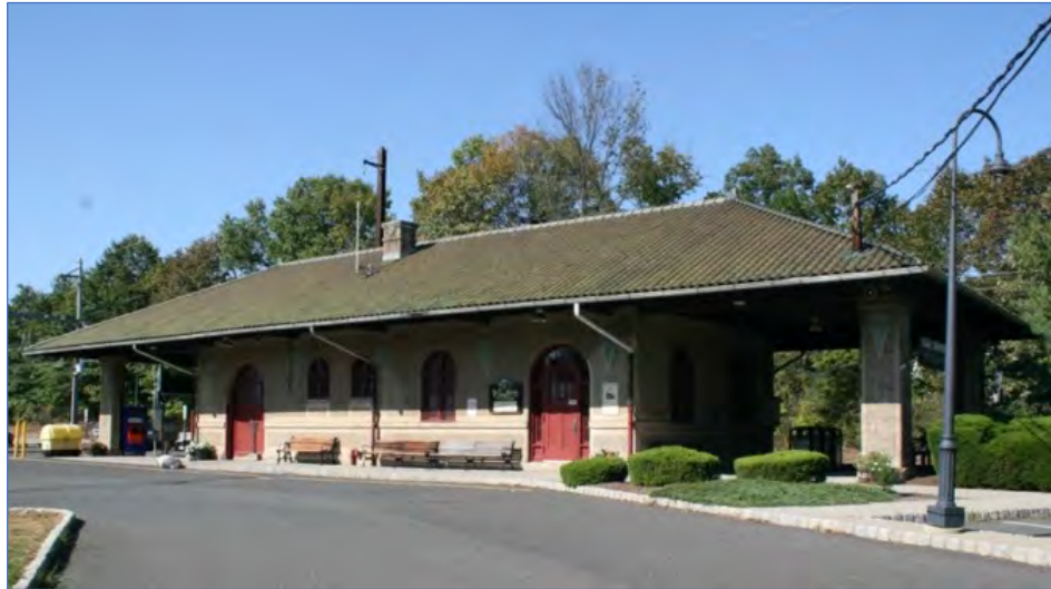
Far Hills Train Station in the Borough of Far Hills. The Renaissance Revival-style station was built in the second decade of the twentieth century of concrete, newly in use by the railroad because of its large-scale need to address extensive track elevation and depression work along the line.
