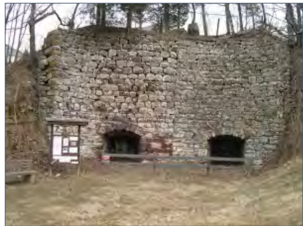
Moses Craig, a farmer in Peapack, joined the manufacture of burnt lime when he built these kilns in 1860 to process the abundant limestone of the area. According to the Historical Society of the Somerset Hills, which received the limekilns as a donation in 1999, "Burnt lime revolutionized and revived northern New Jersey's agriculture in the 19th century." Pulverized limestone replaced burnt lime in the 20th century and the kilns ceased production after 1934. (Photo courtesy VisitSomersetNJ)
