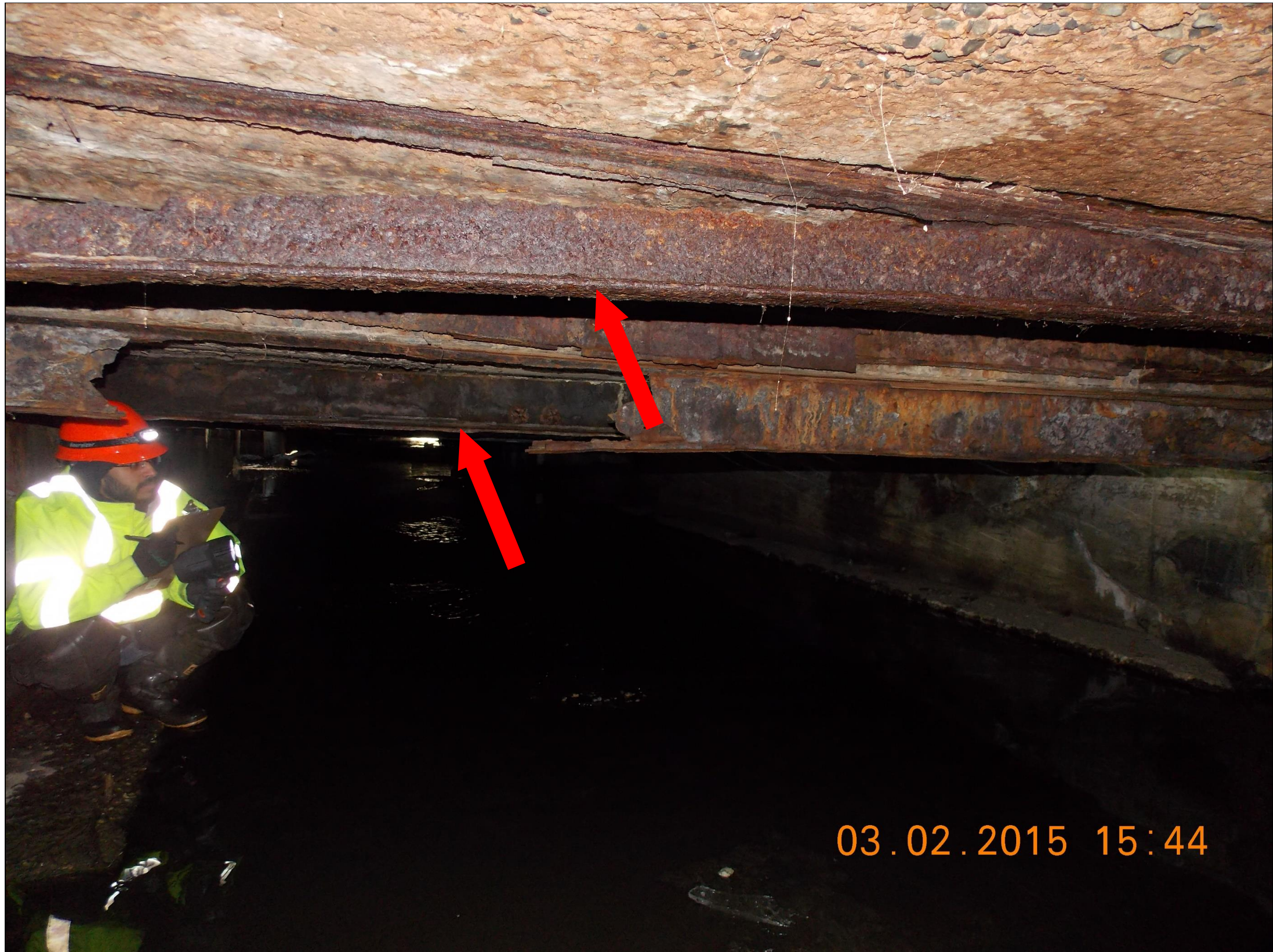
PHOTO 7 M1019 SOMERSET STREET: LOOKING EAST AT LOW CLEARANCE STRUCTURE AND SEVERELY CORRODED STRINGERS
