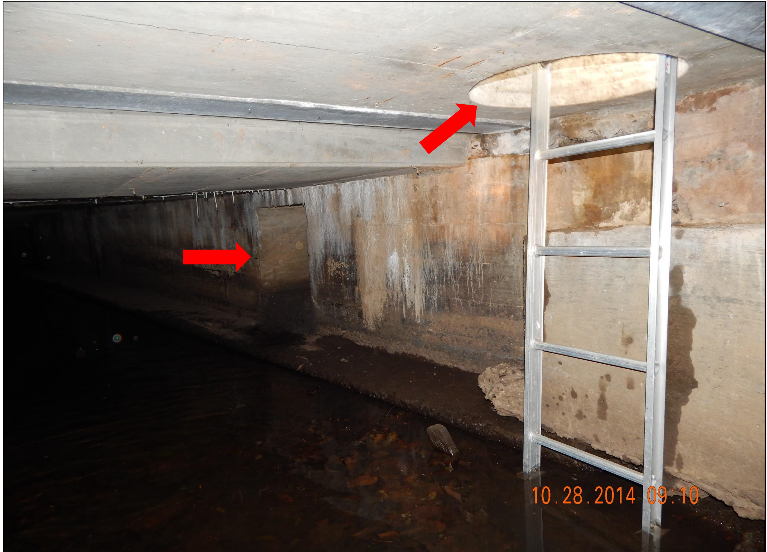
PHOTO 4 M1019 SOMERSET STREET: LOOKING WEST AT ACCESS MANHOLE AND DRAINAGE INLET
