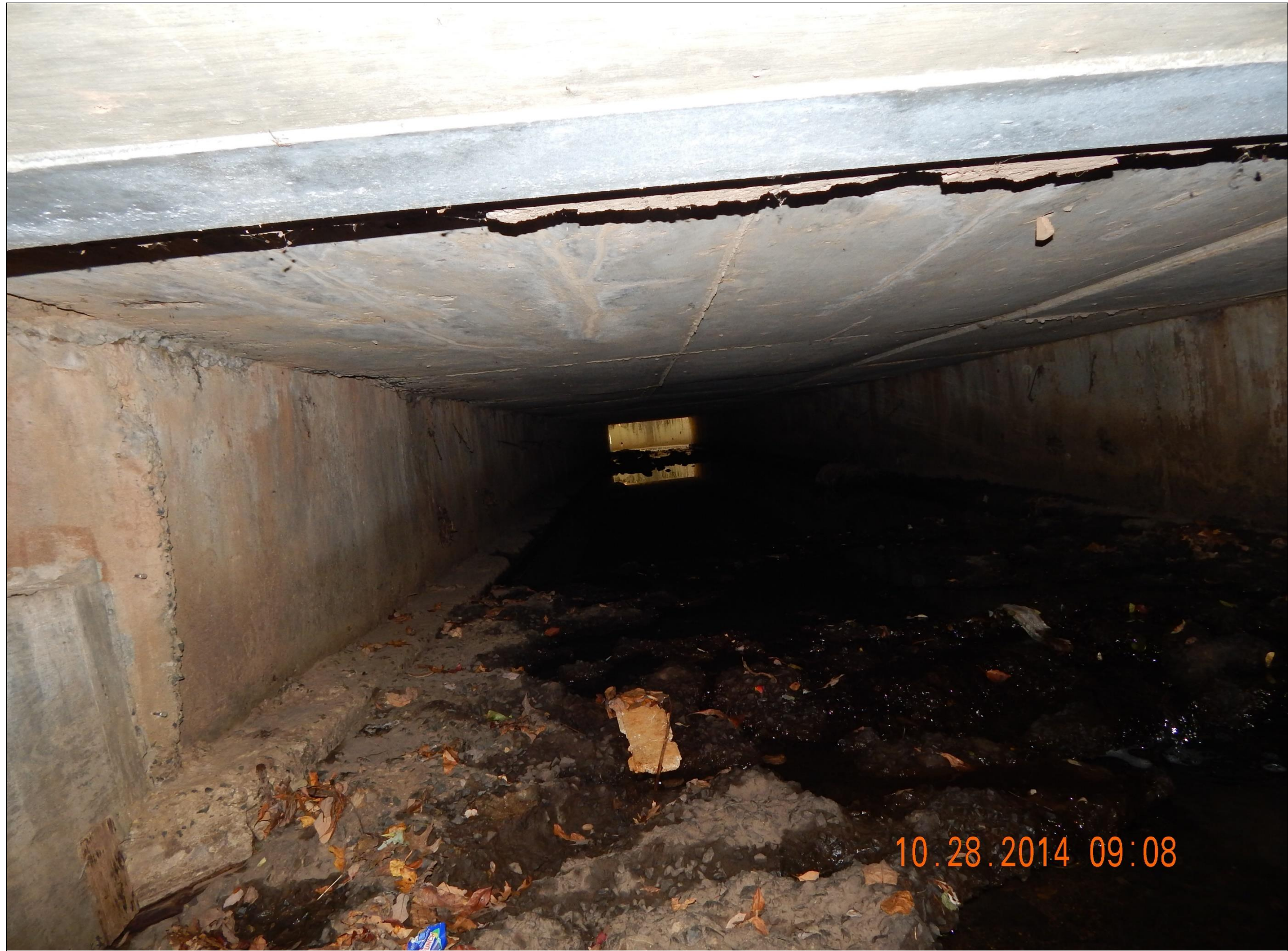
PHOTO 3 M1019 SOMERSET STREET: LOOKING EAST AT ADJACENT UPSTREAM STRUCTURE
