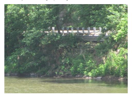
The slope instability has required past pavement repairs and contributes to the poor pavement condition. Temporary repairs made in recent years include replacement to sections of guide rail and the reconstruction of the pavement along the southbound lane. These temporary repairs have allowed the road to remain in use by the traveling public until more extensive permanent improvements can be made to alleviate the ongoing erosion issues along the river.
